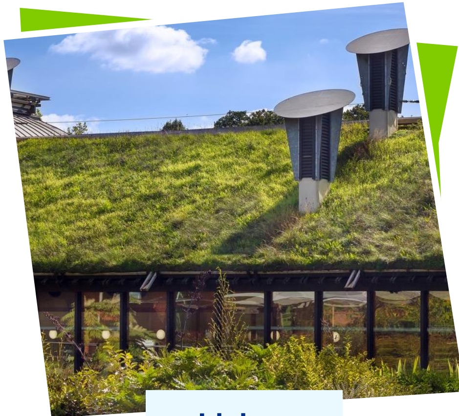
Living, green roof
